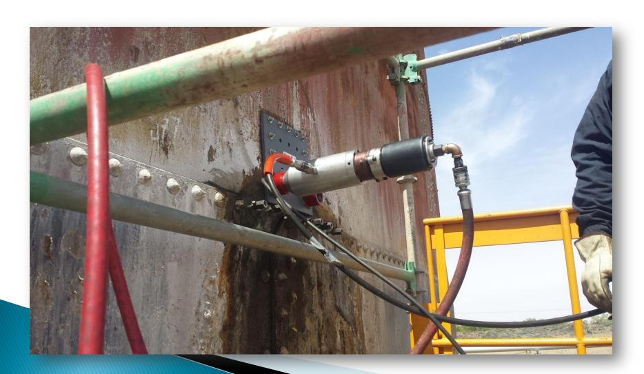
Final Mechanical Repair Plate constructed from 304 stainless steel with a compression gasket with an option to inject as a secondary sealing capability.
