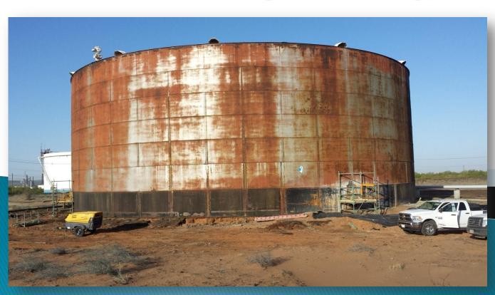
Active external waste water leak between the first and second shell course of a 130 foot diameter in-service tank.
