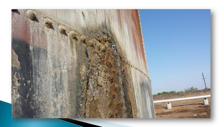
Defective area (crack circled in yellow). Forge Tech Technicians mark stud locations and conduct UT readings for thickness verification.
