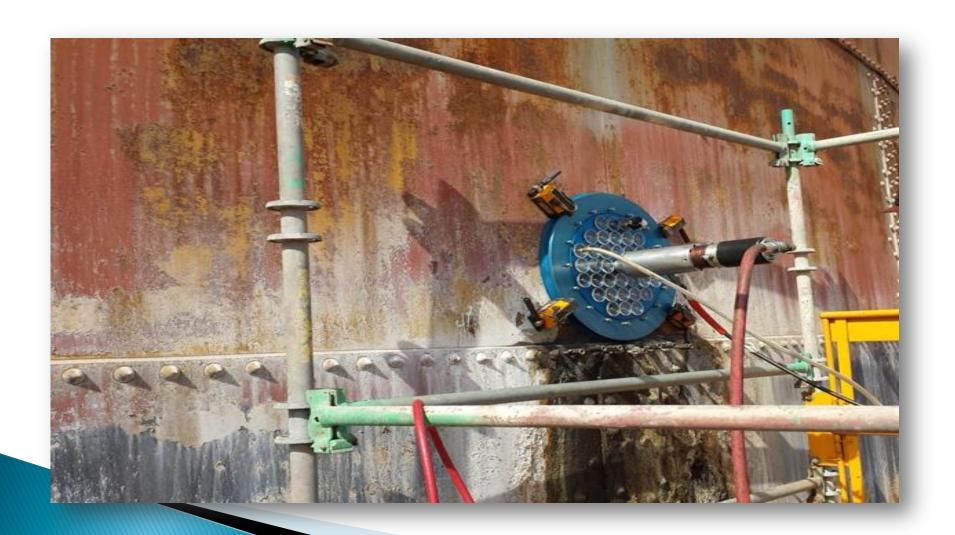
Forge Tech applying Friction Bonded Studs utilizing an Adaptor Plate secured by previously installed studs. The Adaptor Plate allows for locating additional studs as required.
