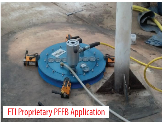
Install Studs Without Hot Work Permit
