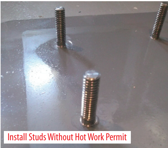
Roof Top Repair on Above Ground Storage Tank
