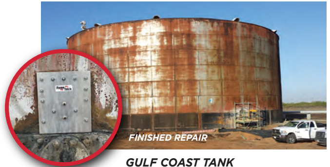
GULF COAST TANK ON-LINE REPAIR
